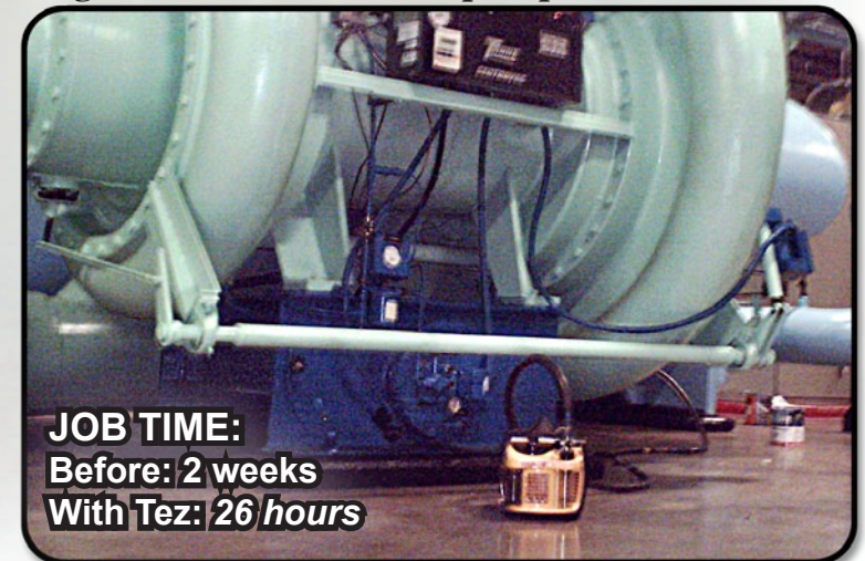
Below: Thanks to massive flow and on-the-fly oil changes, in just 26 hours, the Tez8 evacuated six 1500-ton chillers, one at a time, to 500 microns... outperforming a 20-cfm belt-driven pump.
